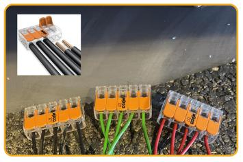
Figure. C.C | 2. Connect wires to terminal blocks
