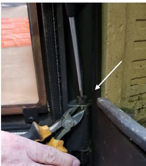
Remove the split and tighten the screw (clockwise) depending on how fast the door should close
